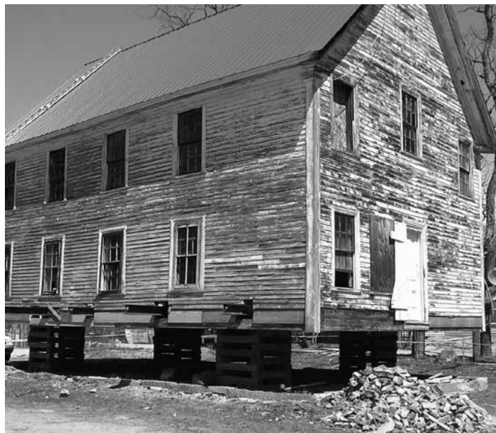
Centennial Hall raised off its foundation during restoration in 2013.
