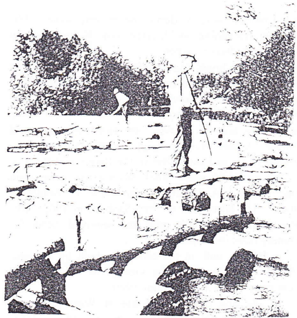
"Slipping logs" through the sluiceway in the old dam, for the use by mills downstream
