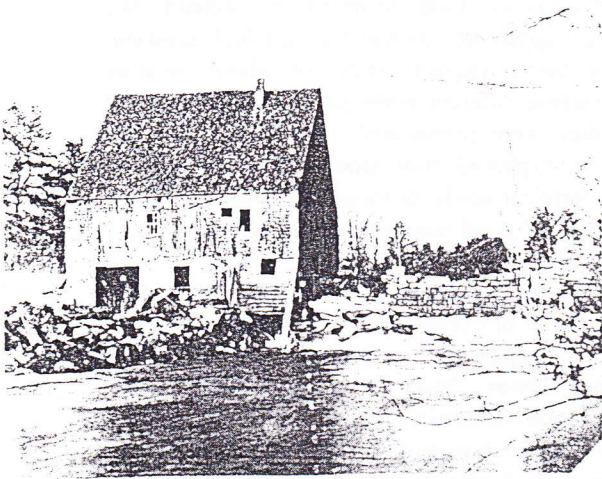
The "Lower Mill" -looking upstream August, 1898
